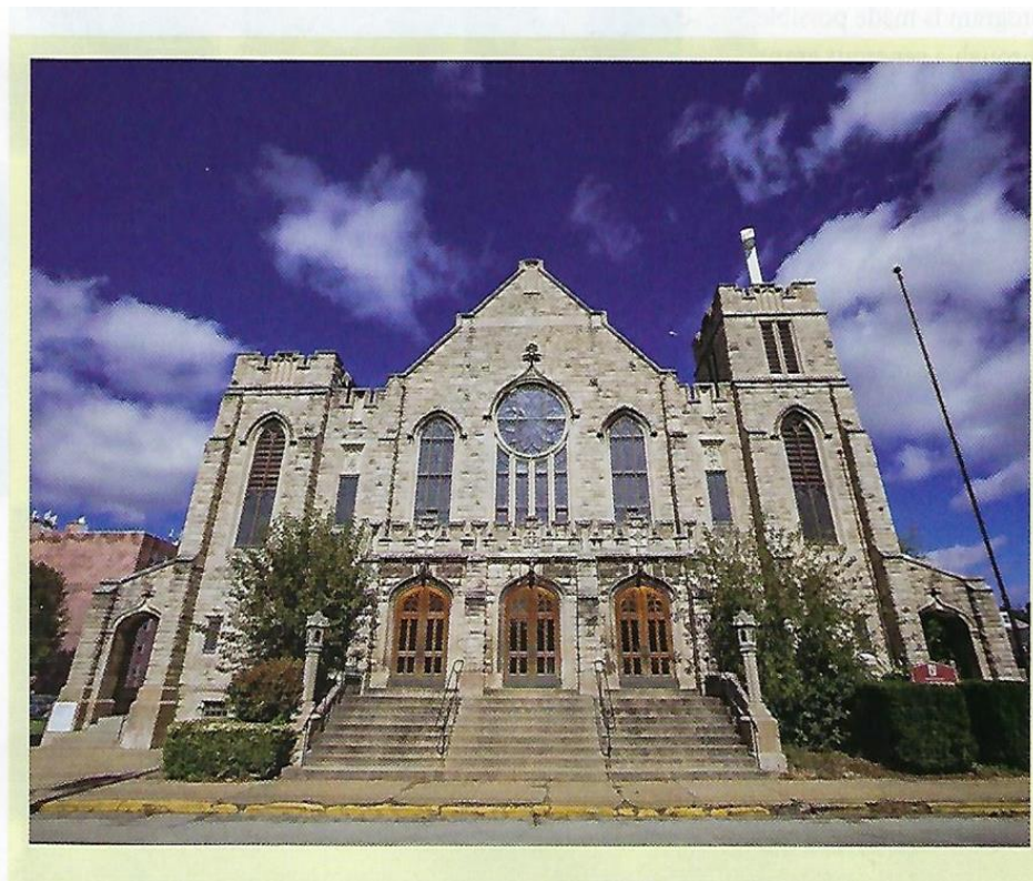
South Avenue United Methodist Church
